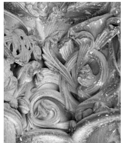
Châlons Notre-Dame W-sR4-5 junction
