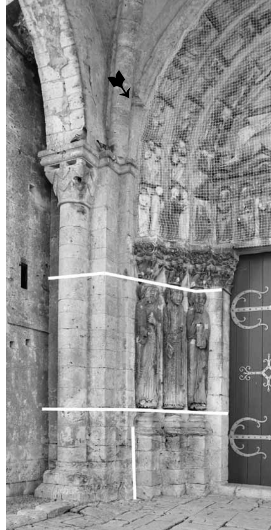
Saint-Loup-de-Naud connections between left embrasure and staircase
