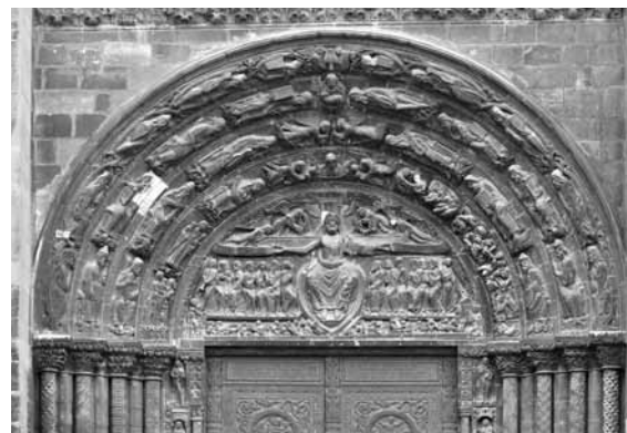
Saint-Denis narthex central portal
