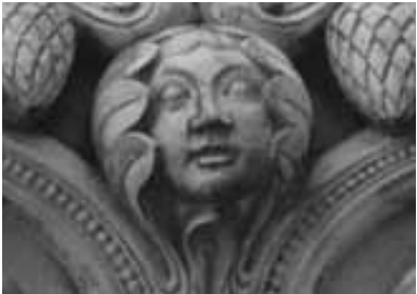
Chartres portal drip W.cL^ (replaced)
