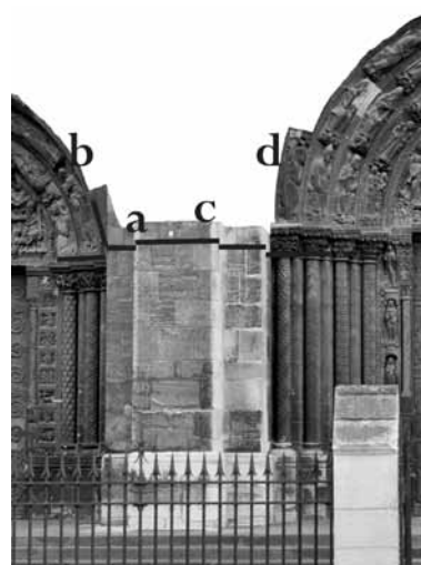
Saint-Denis portal construction detail
